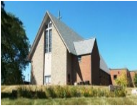
Fellowship Hall Entrance
